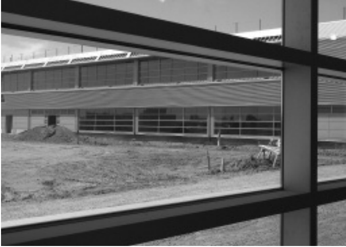
Construction on new Newark Campus. Photo courtesy of College Relations.
