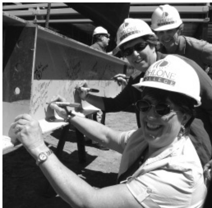
Vice President Jim Wright, Associate Vice President Leta Stagnaro, and Dean Mikelyn Stacey sign the last beam to be set in place in the construction of the Newark Center for Health Sciences and Technology. Photo courtesy of College Relations.
