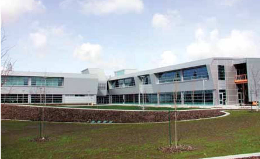
Ohlone College Newark Center for Health Sciences and Technology Campus is the nation's first "green" community college campus.
