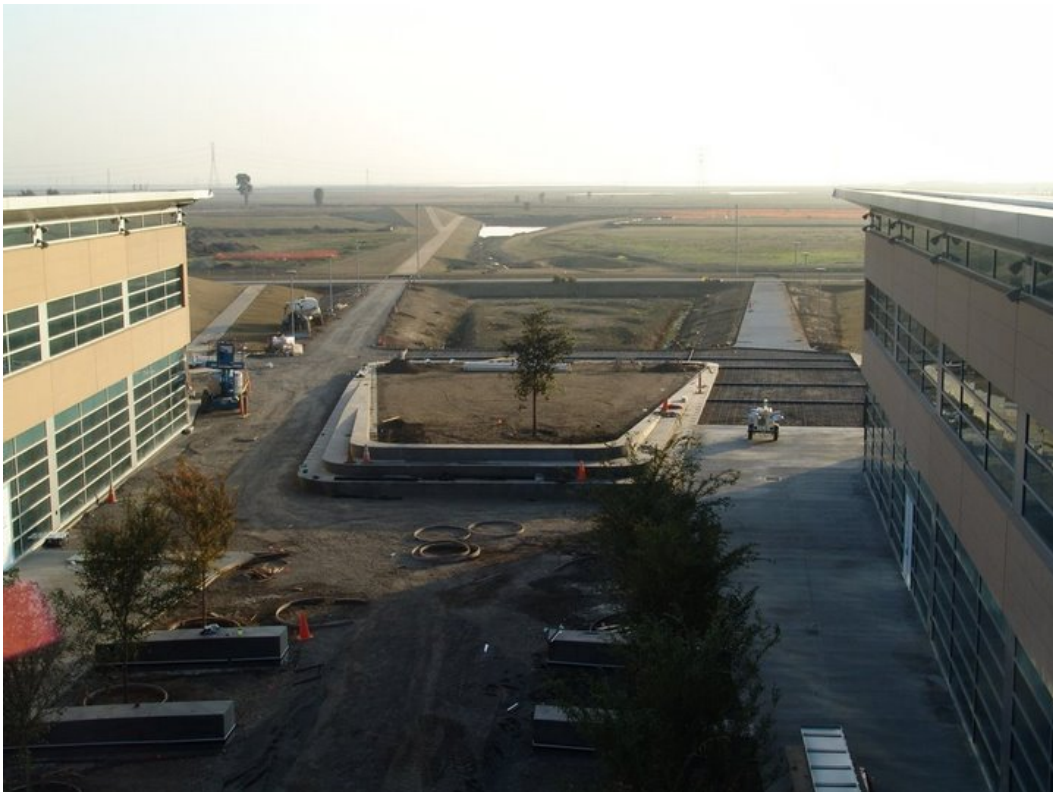
View of site during construction in the Southern direction
