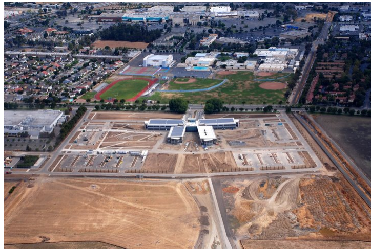
Aerial view of the project during construction
