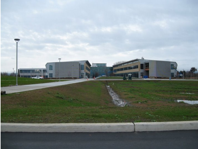
Stormwater garden during low-flow event
