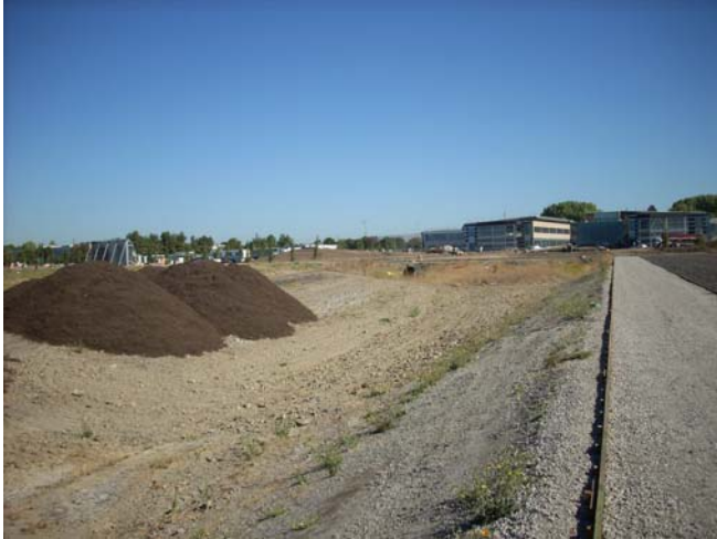
Views of the stormwater swale/retention pond prior to hydroseeding
