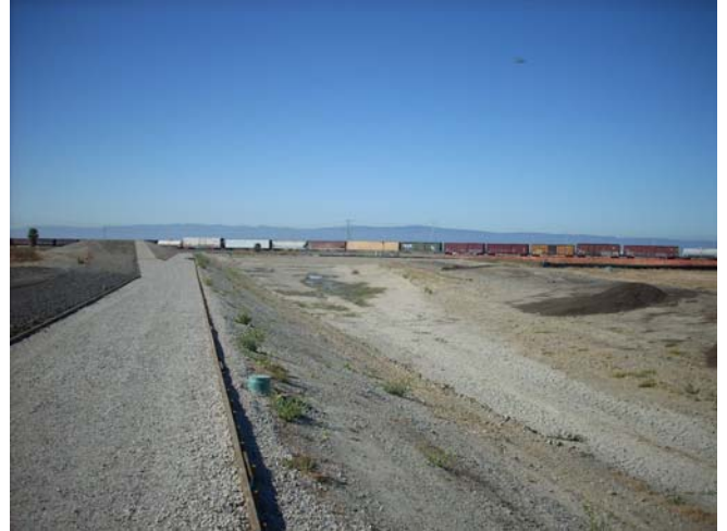
Views of the stormwater swale/retention pond prior to hydroseeding
